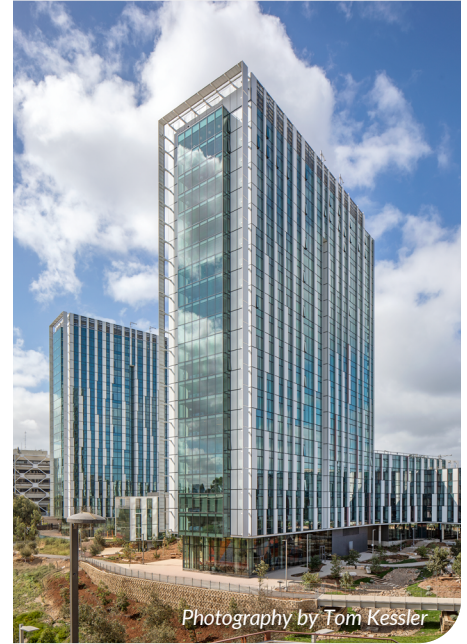
Perforated metal shading fins were strategically installed throughout the Solarban® glass façades to create a peeling bark aesthetic and minimize solar heat gain.
